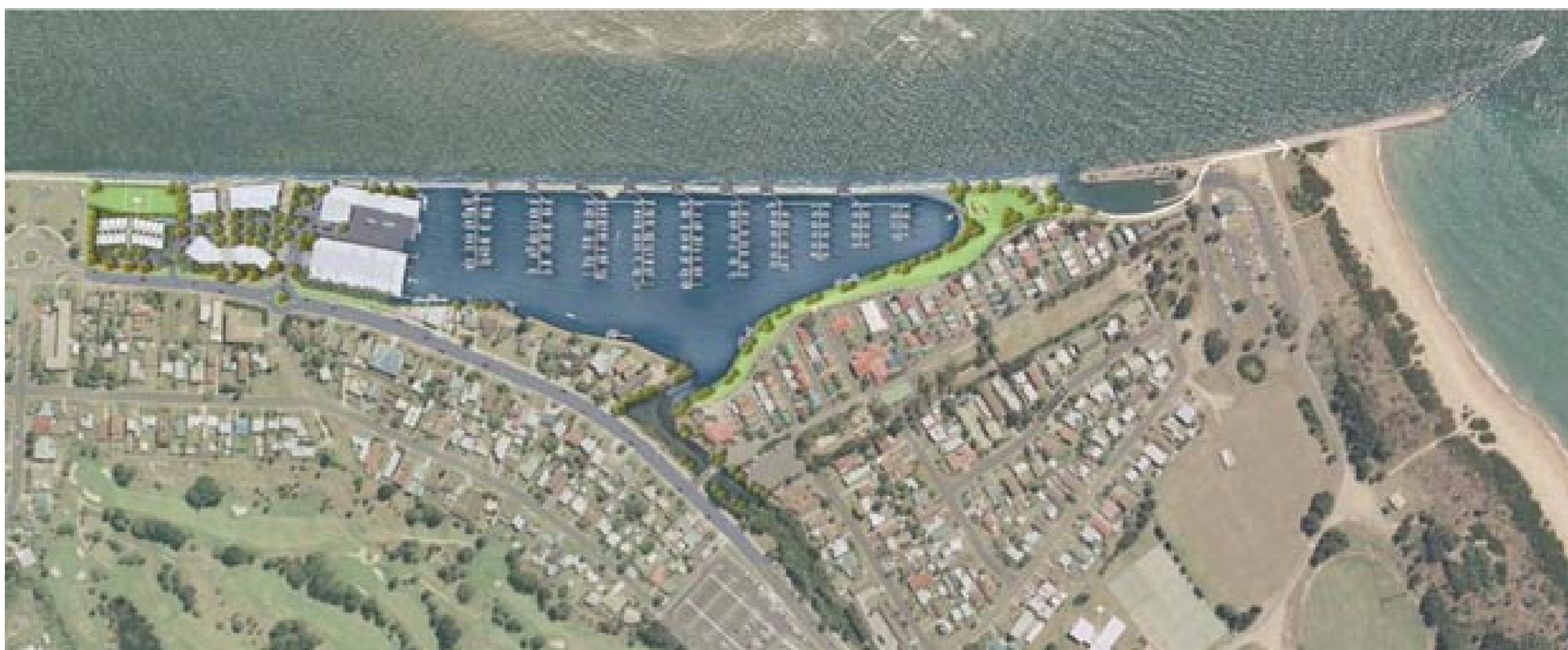
Top: Aerial view of the current Marina Bottom: Artists perspective of the redeveloped Batemans Bay Marina
