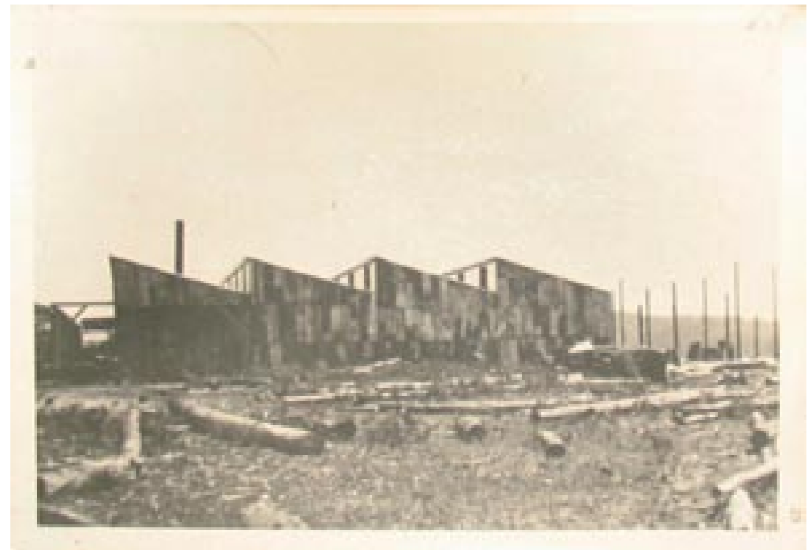
Historical Batemans Bay Shed - Perrys Mill 1903 facade patterning
